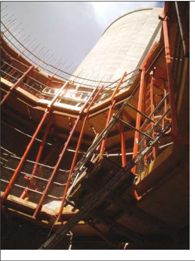
Figure 3. Inside the slipform for the lime silo.
