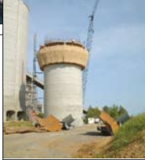
Figure 7 (right). Construction of the new lime silo.
